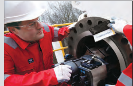
▲ Flange facing machines to ensure flange joint integrity.
