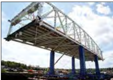
Incremental bridge lifting
