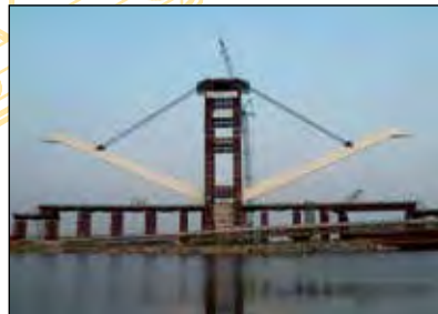
Jacking with high capacity precision control
