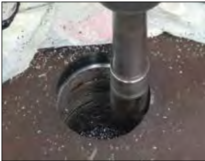
▲ Enlarging a hole
