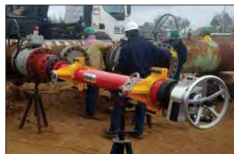
▲ CHT3000 hot tapping application for petrochemical pipeline installation.
