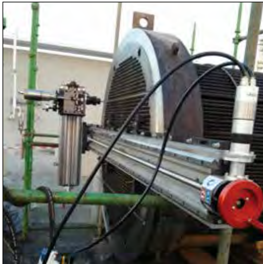
▼ MRY Milling machine on a heat exchanger.
