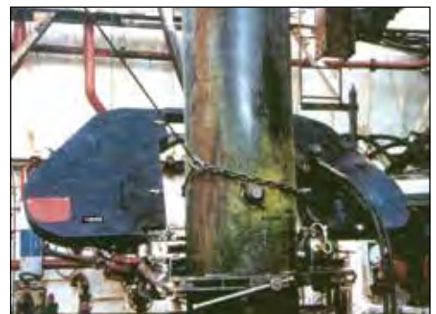
▼ Decommissioning job with band saw.
