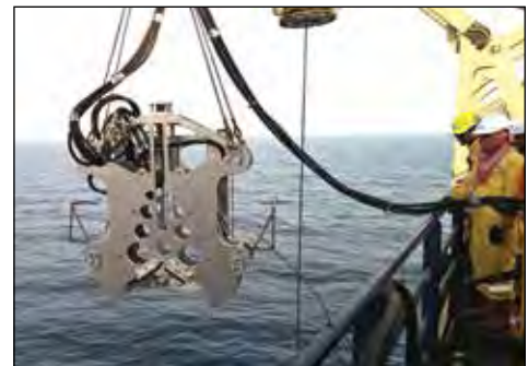
▲ MDWS Diamond Wire Saw lowered into sea.
