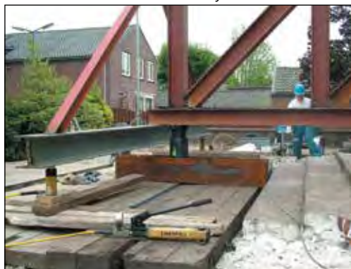
▼ P392 in action with RC256 cylinders.
