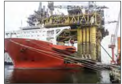
Synchronous superlift and launch
