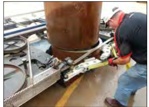
▲ Pipe cutting with BS portable band saw.
