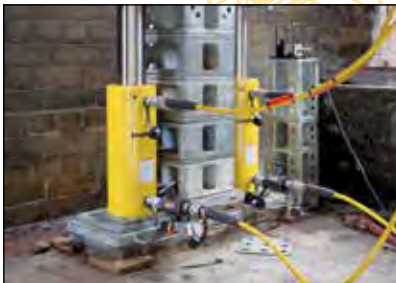
Bridge lifting and launching
