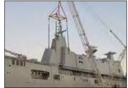
Synchronous hoisting and load positioning
