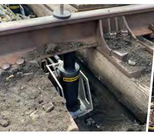
The TL248 Track Lift System includes four framed lifting cylinders, each rated for 62 tons, offering a total lifting capacity of 248 tons.
